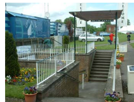
Fig. 42 Steps across Racecourse Road
