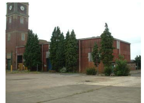
Fig. 3 Later extension to Boiler House
