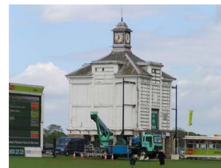
Fig. 30 The abandoned Indicator Board
