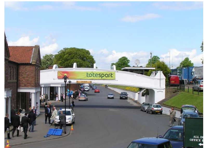
Fig. 35 Bridge link across Racecourse Road
