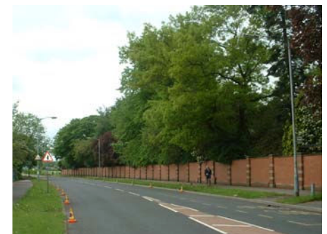
Fig. 6 Existing eastern boundary along Bishopthorpe Road
