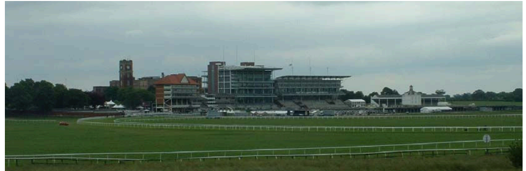
Fig. 10 Conservation Area from west
