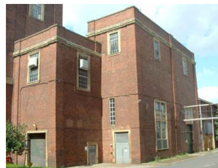
Fig. 53 Boiler and Transformer house
